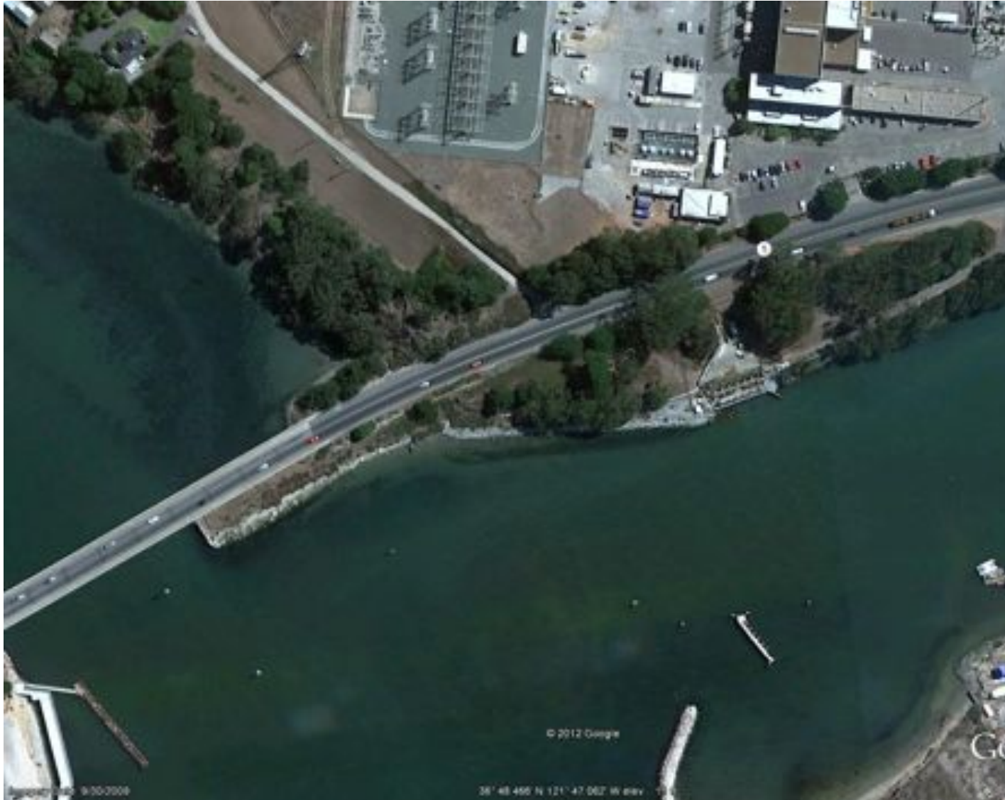
Figure 3. Overview of the area of the abandoned fuel oil pipeline near the Moss Landing Power Plant.
