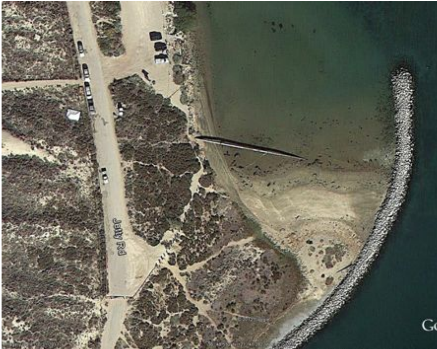
Figure 2. Close up of the abandoned fuel oil pipeline near Jetty Road.
