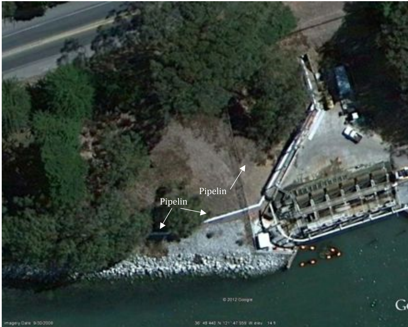
Figure 5 Continuation of the abandoned fuel oil pipeline near Moss Landing Units 1 & 2 Intake Structure. See overview in Figure 3.
