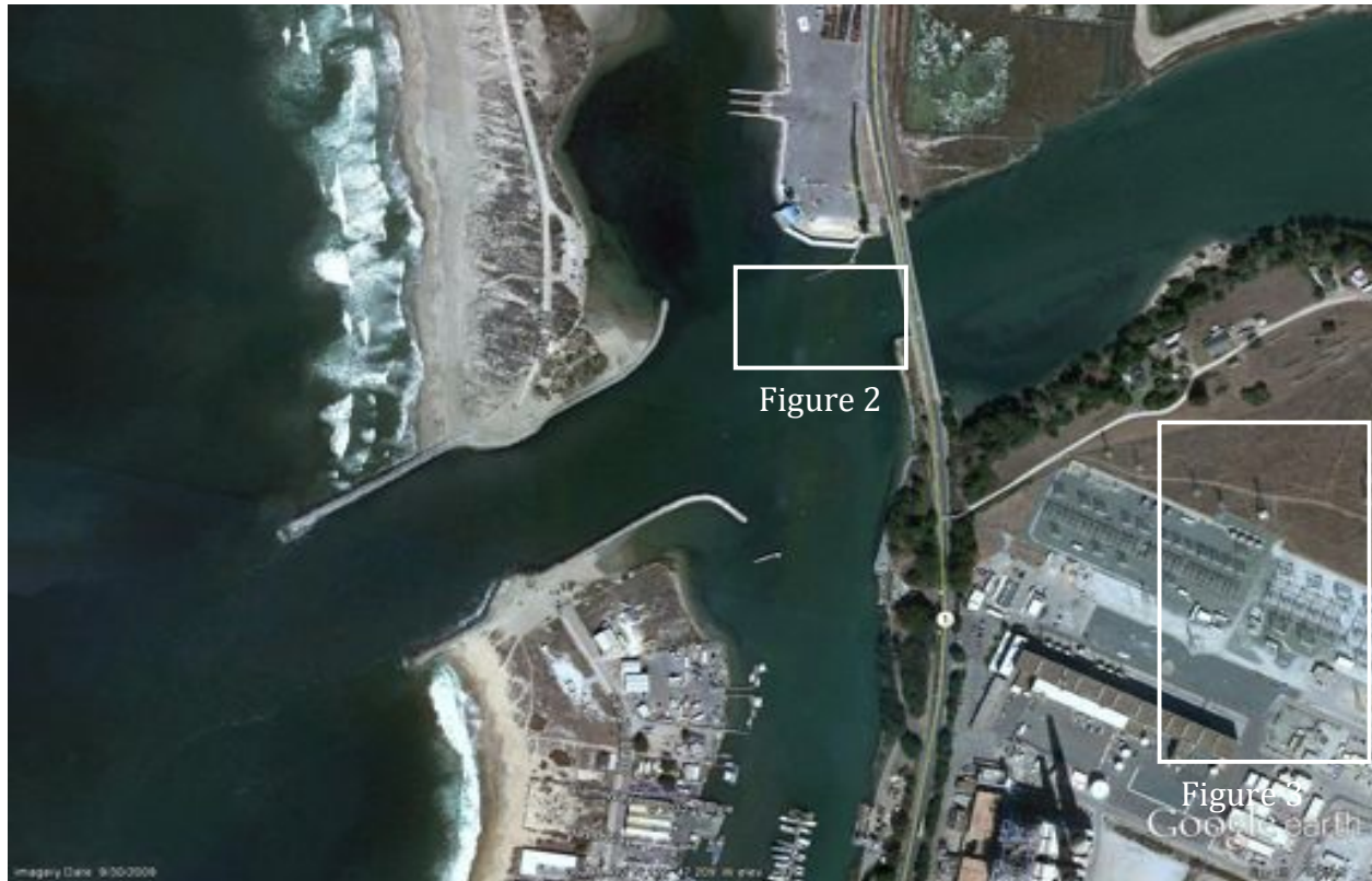
Figure 1. Overview of the area showing Monterey Bay, Elkhorn Slough, Moss Landing Harbor, Highway 1 Bridge, and the Moss Landing Power Plant. The abandoned pipeline is first seen inside the box marked Figure 2 (see following Figure 2 for a close-up view). The pipeline can be seen again inside the box marked Figure 3 (see following Figures 3–6 for close-up views).
