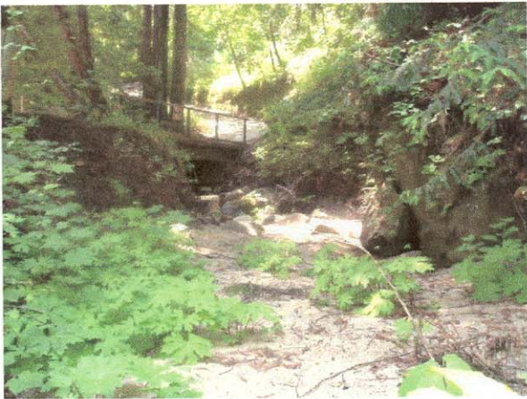
Picture 3 Downstream side of first new bridge
