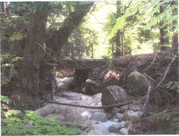
Picture 2 Upstream side of first new bridge
