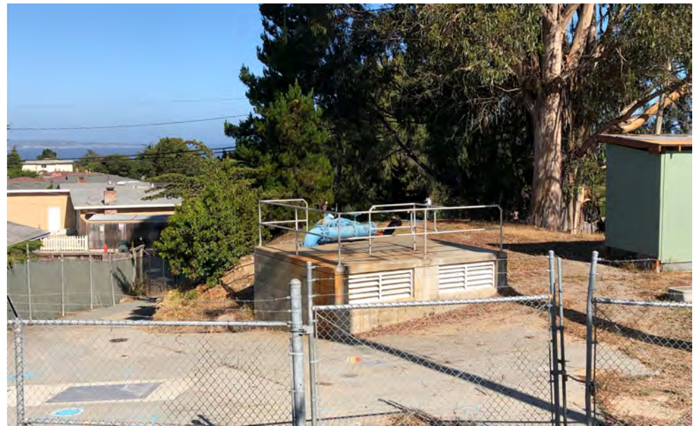
Photo 2. Proposed de-chlorination facility facing west.
