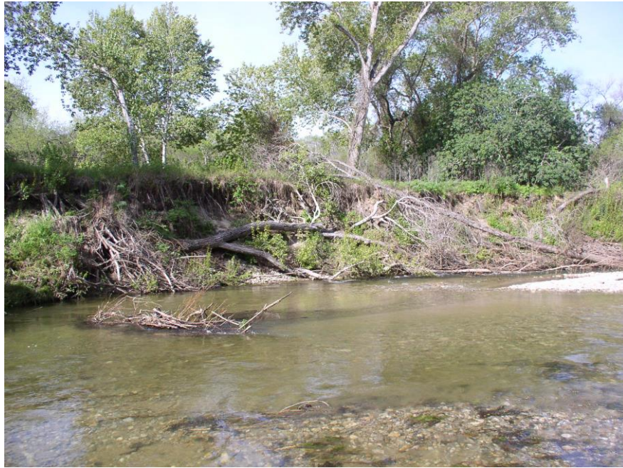
Left Bank Looking Downstream before Bank Stabilization (Spring 2017)
