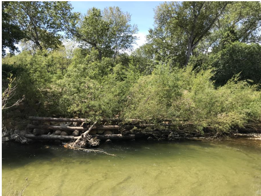
Left Bank Looking Downstream after Bank Stabilization (April 2023)
